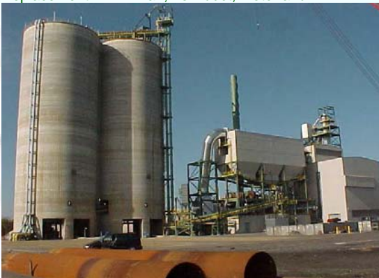
Slag grinding facility 2x10000 MT
