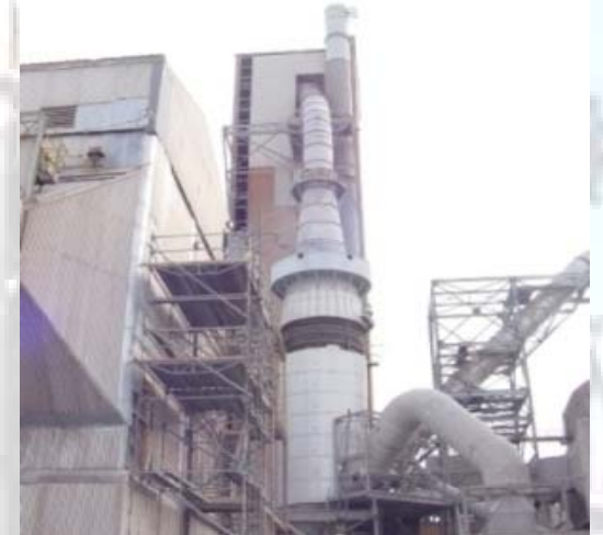
Gas conditioning tower upgrade & new P/H duct
