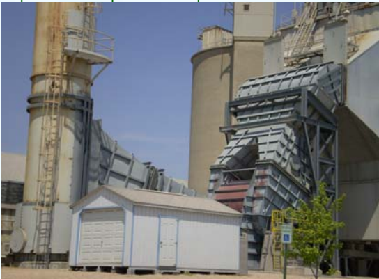
Replacement kiln ID Fan, new duct, motor and VFD
