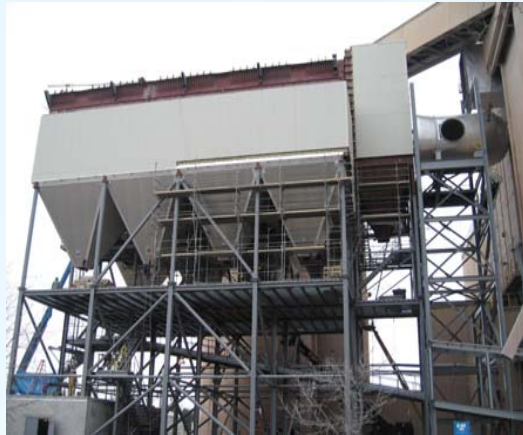
800,000ACMH/RM pulse jet BH to replace EP
