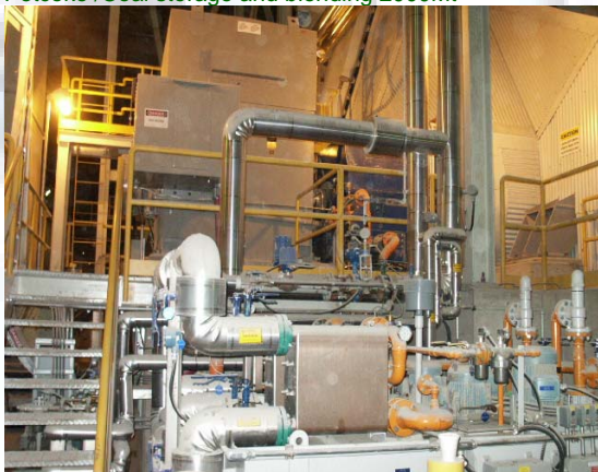
5000hp Synch motor with Fluid Coupling, P/H ID fan
