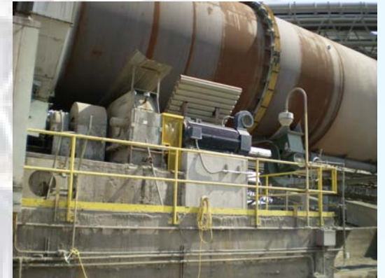
New kiln drive retrofit 2x300 hp, long dry kiln
