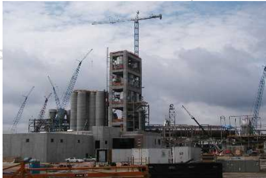
6000 TPD Preheater concrete tower
