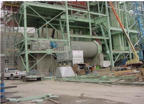
120 TPH Cement Ball mill
