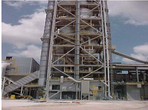
2200 TPD steel preheater tower
