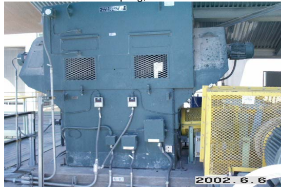
1100 kW, 1800rpm, 4.16 kV, kiln drive motor & VFD Please visit our WEBSITE or contact us at:
